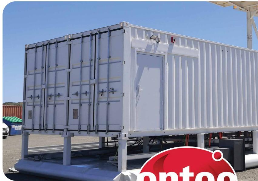
A PREFABRICATED PLANT ROOM: BUILT OFF SITE
